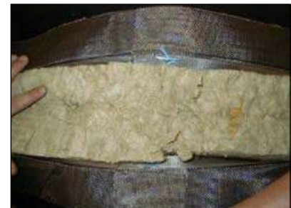
6. Butt Insulation Over Splice
