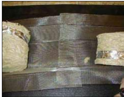
2. Fold Back Insulation and Overlap
