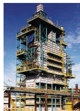
Ethylene Cracker Unit
