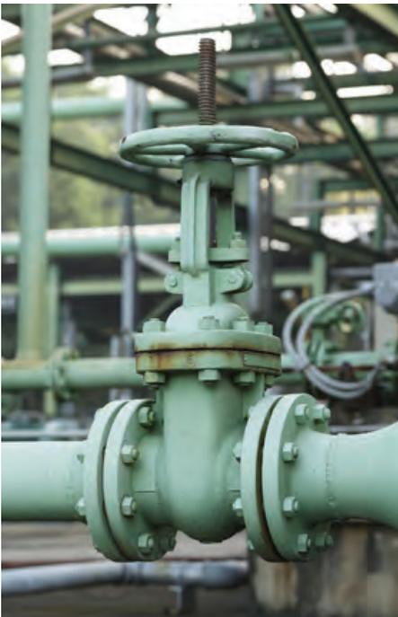
Basic to all power generation facilities is their extensive piping systems. Flange gasketing, while not a large part of the overall expense of the system, is however very important to the continued operation and safety of the workers in the environment.
