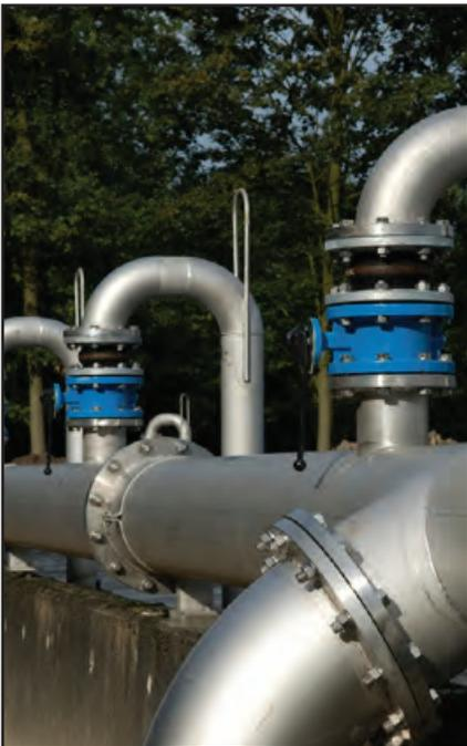
Piping systems require proper layout, support systems and equipment to handle vibration, misalignment, and transitions. Elastomeric expansion joints are a critical component in these systems, allowing for thermal movement, vibration and correcting misalignment.
